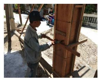
Fig. 12 One of the builders used hummer to compact the placed concrete
