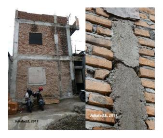
Fig. 13 Sample of structural defect due to improper compaction
