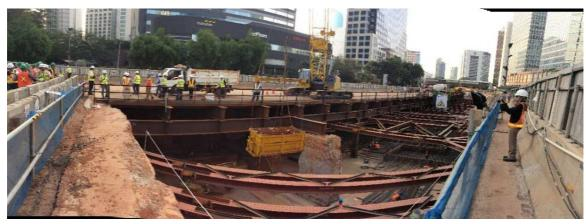
Fig. 11 Top down construction method to reduce traffic disturbance
