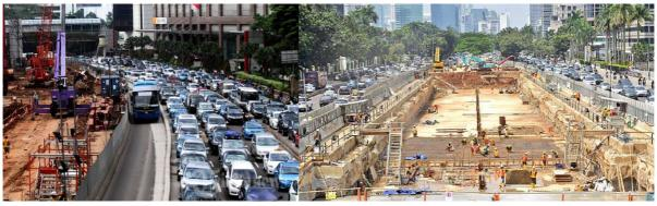
Fig. 8 Managing the traffic flow around the excavation in the North Corridor
