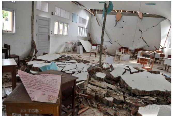
Fig. 9 Failures of school due to high amplification of seismic ground motion inducing foundation failure.
