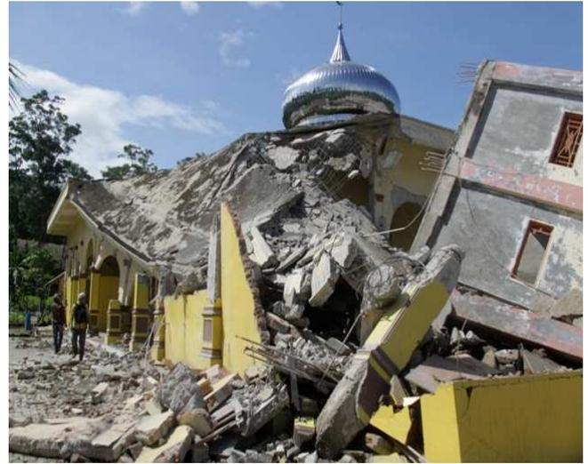
Fig. 8 Failures of vulnerable mosque due to high amplification of seismic ground motion inducing foundation failure.
