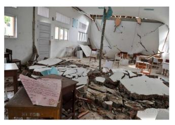
Fig. 9 Failures of school due to high amplification of seismic ground motion inducing foundation failure.
