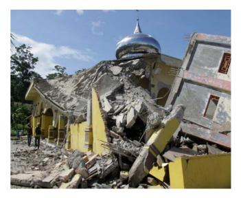
Fig. 8 Failures of vulnerable mosque due to high amplification of seismic ground motion inducing foundation failure.
