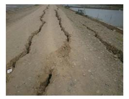
Fig. 11. Ground failure in Manohara-shorelines Pidie Jaya Aceh earthquake 7th December 2016.
