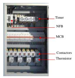
Fig. 8 Aeration control module
