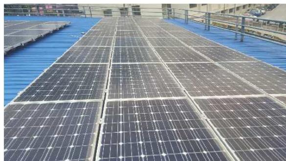
Fig. 1 Monocrystalline PV array (System 1)
