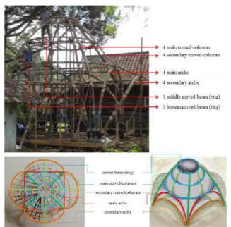
Fig. 9 Curved structural elements
