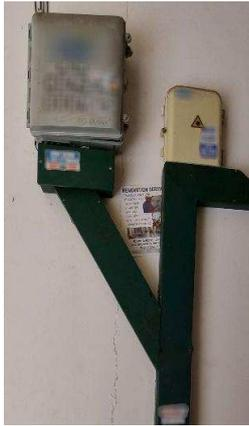
Fig. 1 A sample of indoor Fiber Distribution Panel box installation. Some parts are blurred out due to confidentiality concerns.
