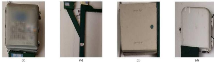
Fig. 3 Sample illustration of (a) FDP box, (b) green trunking, (c) copper box and (d) fiber box. Some parts are blurred out due to confidentiality concerns.
