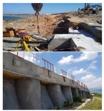
Fig. 7 Treatment by the use of piles anchor for some cases of Al-Ghandouri landslides
