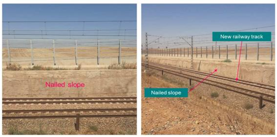
Fig. 11 Nailed slope and new railway track
