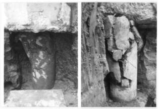
(b) Hyogoken-nanbu (Kobe) earthquake 1995 Fig. 1 Spun pile damage after the earthquake [1],[2]
